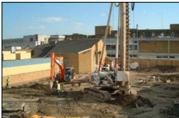
CFA piling rig
