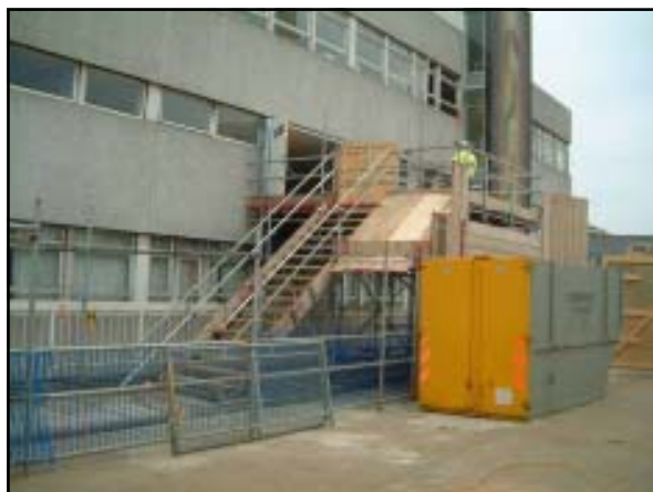
Construction access to the Endoscopy Suite
