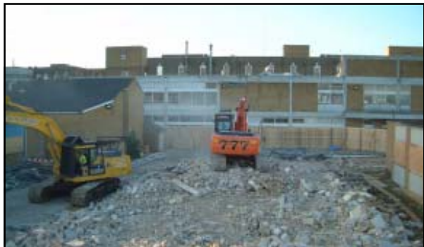
The saw cut existing concrete slab being removed
