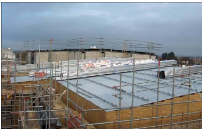
Ward Roofing's standing seam roof with traditional eaves detail
