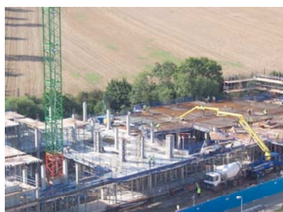
New building under construction
