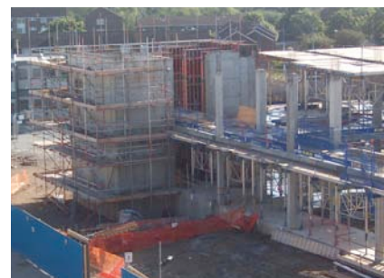
New building under construction
