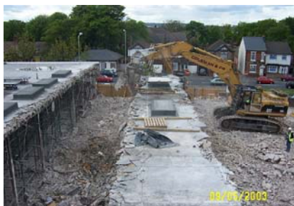
Controlled Demolition in Progress Adjacent Live Departments
