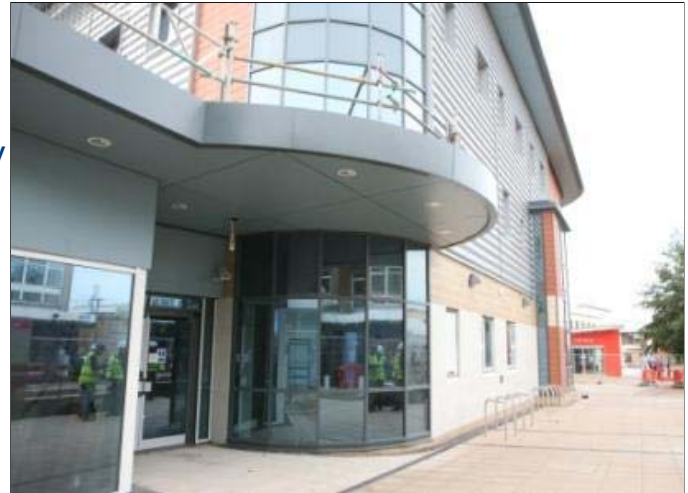
The Yate Health and Children’s Centre in Yate town centre – Shortly before completion
